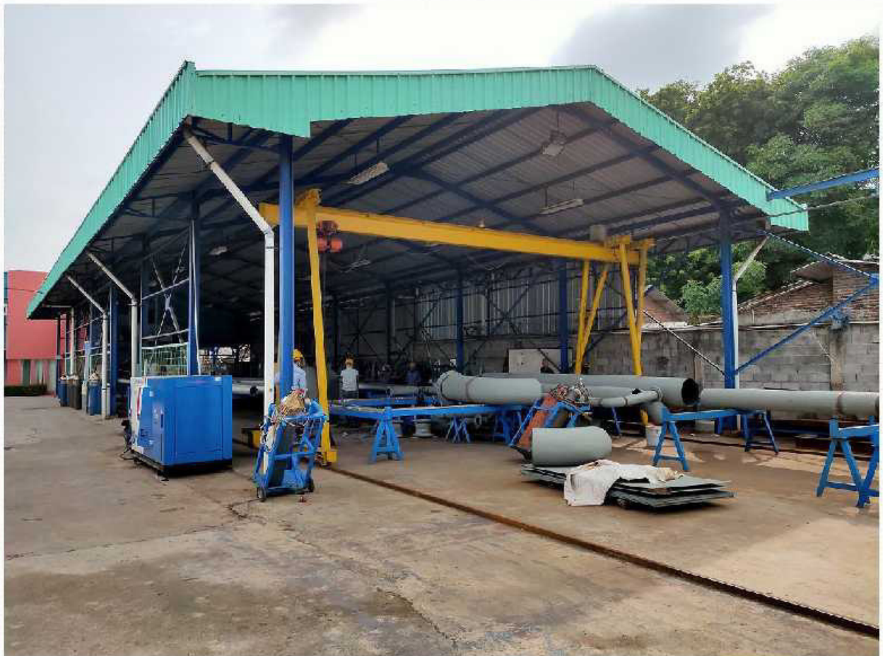
WORKSHOP BUILDING PT SAHAMI TEKNINDO UTAMA
