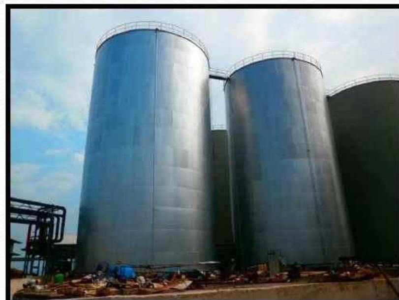
FABRICATION & ERECTION TANK 3000 MT
