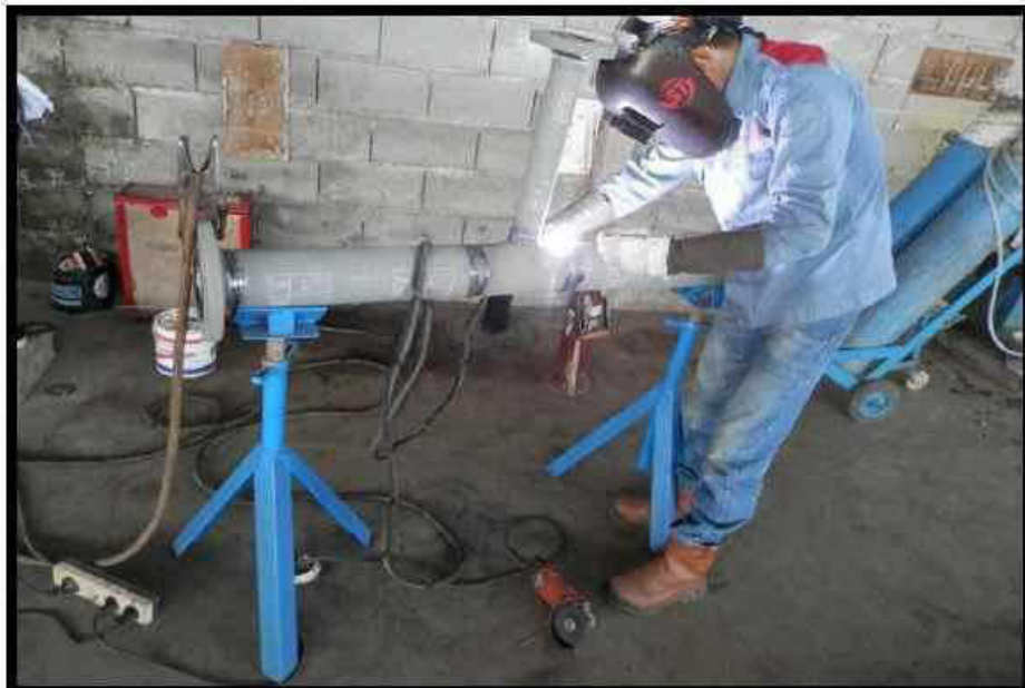
PIPING FABRICATION AT WORKSHOP PT. STU
